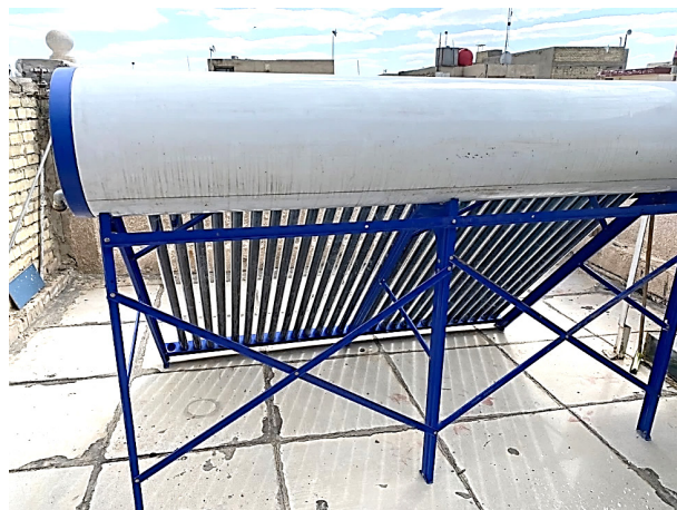
Figure 4. Tilt solar collector
