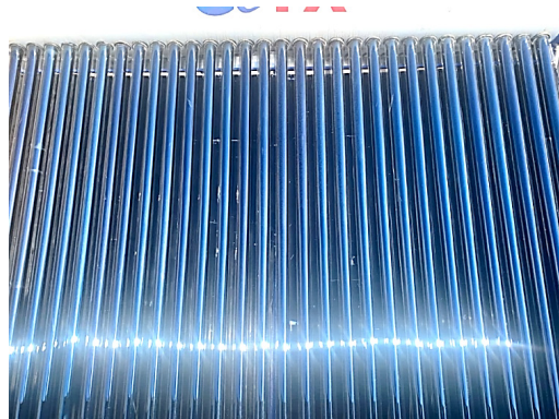
Figure 2. Evacuated tubes
