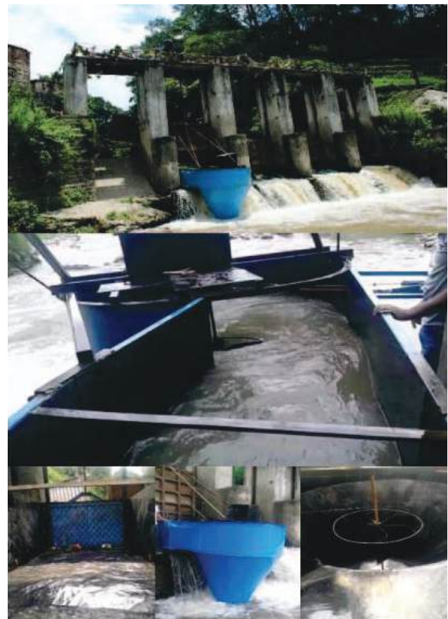
Figure 17. This project is a test run for a conical basin design incorporating a runner, intake canal, irrigation canal weir, and basin construction.
