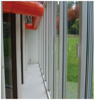
Figure 4. Buffer space with indirect gain.
