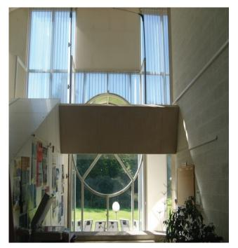
Figure 3. Central zone with direct gain.
