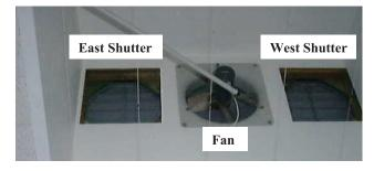
Figure 5. Heat extractor system.
