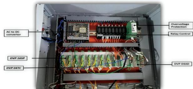
Figure 6. Construction layout of hardware in NMDAS.
