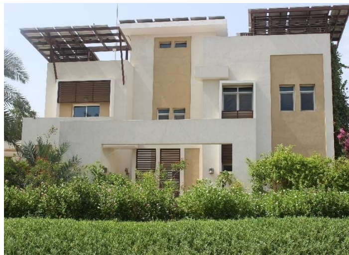
Figure 1. Net-zero energy building at higher college of technology Muscat
